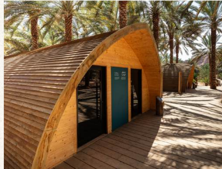
Daimumah wooden eco-lodge - Daimumah in the Cultural Oasis
